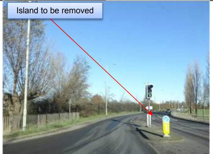
8.4.6.4. – View on junction
