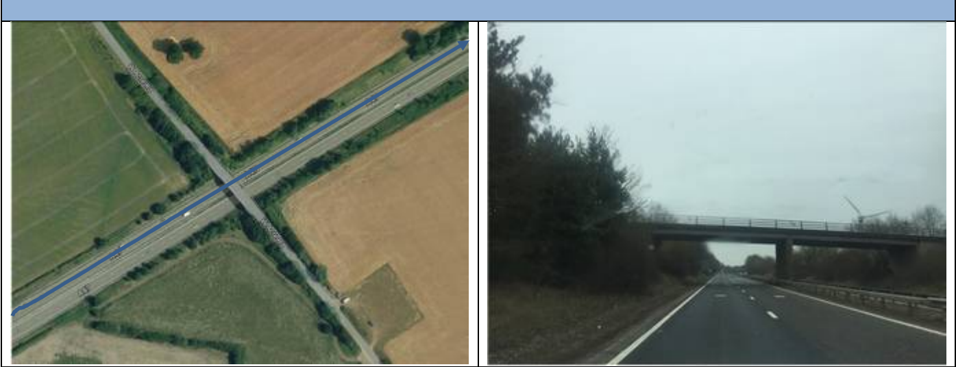
8.8.2.1. – Aerial View of Location | 8.8.2.2. – Reverse view of bend
