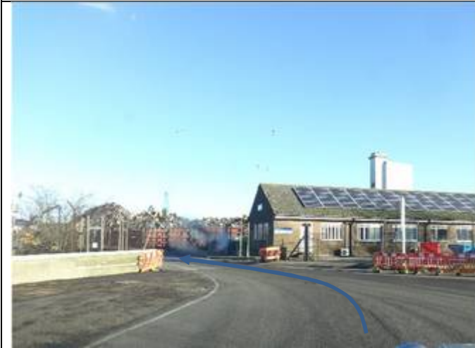
8.4.1.3. – View at crossing
